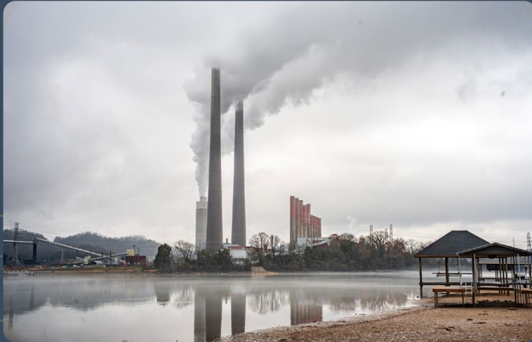
Above: The Tennessee Valley Authority's Kingston Fossil Plant is one of the utility's dirtiest, least reliable, and most expensive power plants, as well as the site of a devastating coal ash spill in 2008. Photo by Abby Hassler
