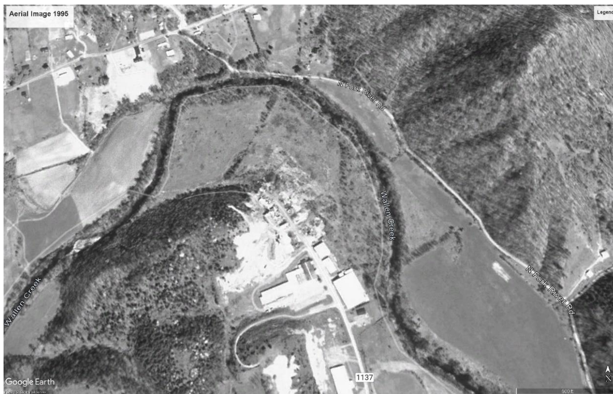
Figure 3. Google Earth Pro Aerial Image from 1995 showing much less vegetation than currently exists and some linear features.
