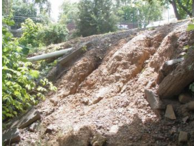
BEFORE: Runoff from Parking Causing Erosion on Streambank
