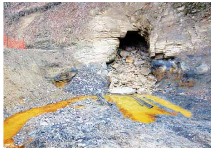
Acid mine drainage at an abandoned mine portal. Photo courtesy of Virginia Department of Mines, Minerals and Energy
