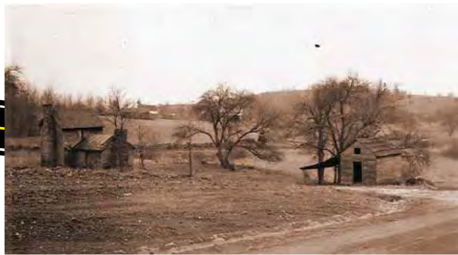
This photograph taken by Robert G. Hall on March 28, 1939, near Swannanoa, N.C., shows abandoned farmland buildings scheduled for demolition to clear a path for the Blue Ridge Parkway. Courtesy of the National Park Service, Blue Ridge Parkway
