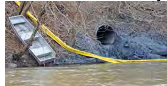
When a Duke Energy coal ash pond failed in 2014, waste entered the Dan River through this pipe. Photo by Appalachian Voices
