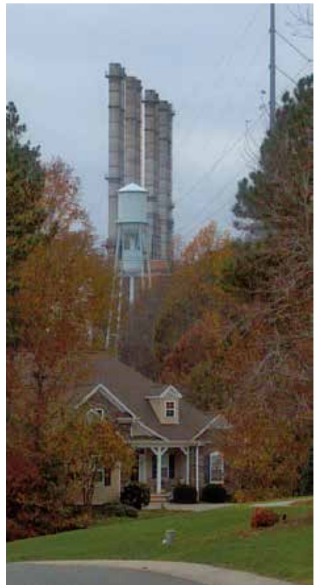
Duke Energy’s Riverbend Steam Plant in Gaston County, N.C., was retired in April 2013; the utility said the plant, which began operating in 1929, was rarely used. Political analysts suggest that outlining a strong plan for reducing its own carbon emissions could give the United States added leverage at the 2015 international climate change conference in Paris. Photo by Sandra Diaz
