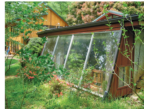
Recycled blue jean scraps provide safe and effective insulation for the Sweet Gum Gateway, left. Above, a window into energy efficiency: the south-facing greenhouse soaks up the sun while the earthen side-walls provide insulation. Photos by Patrick Ironwood.
