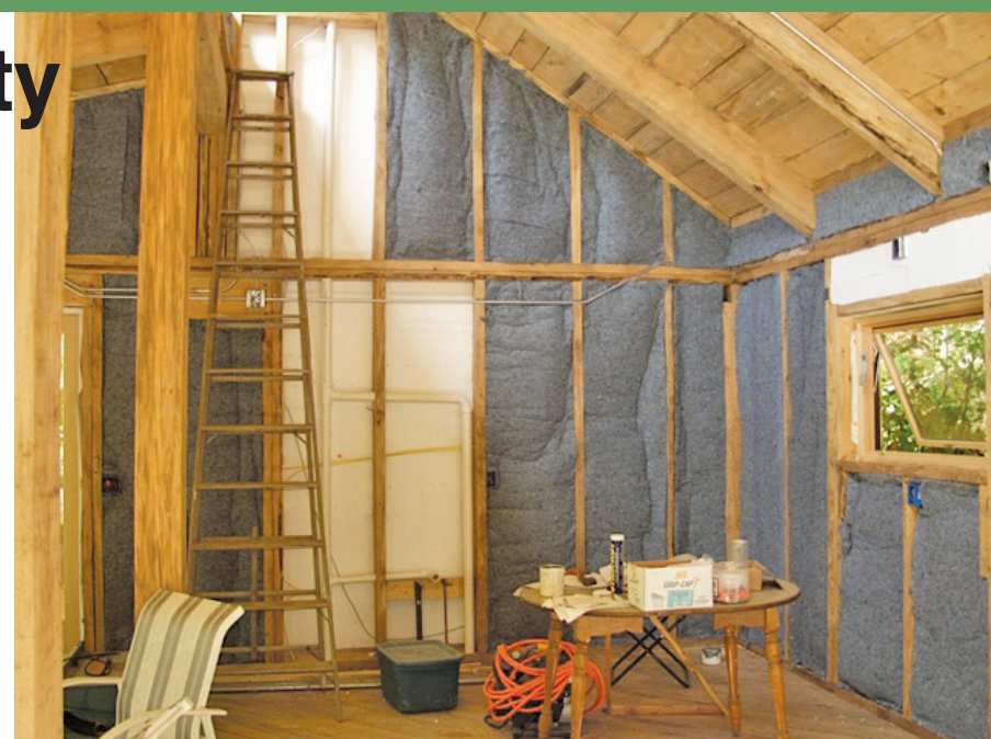
Recycled blue jean scraps provide safe and effective insulation for the Sweet Gum Gateway, left. Above, a window into energy efficiency: the south-facing greenhouse soaks up the sun while the earthen side-walls provide insulation. Photos by Patrick Ironwood.
