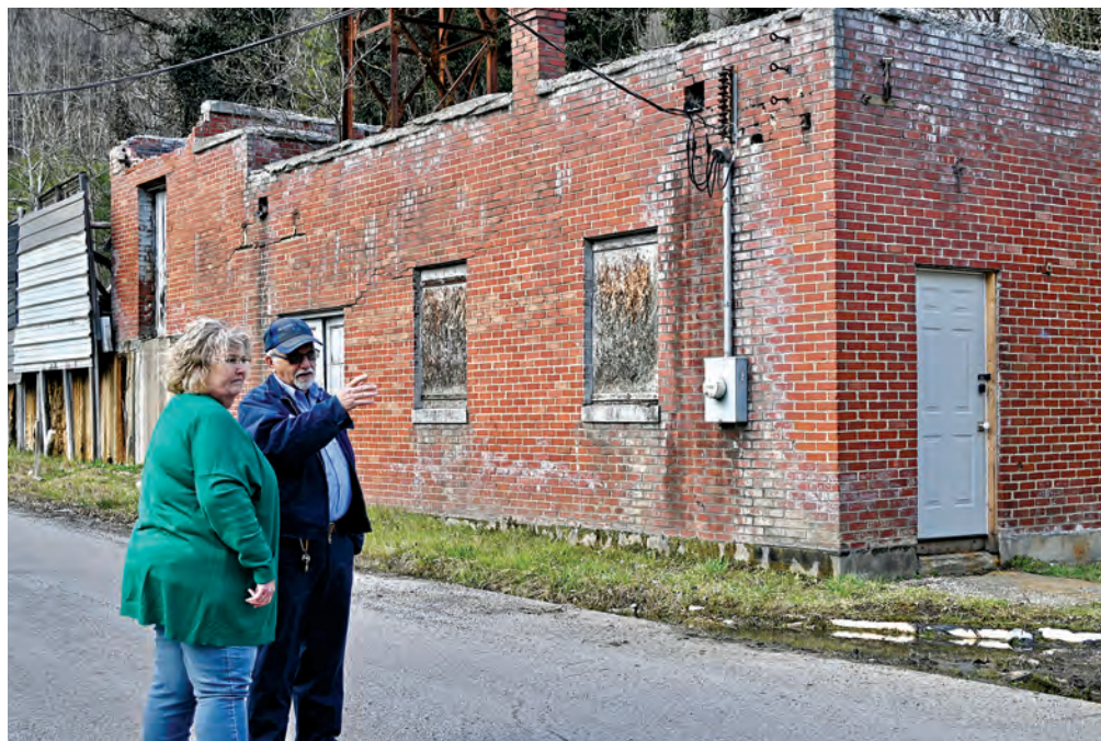
Mavis Brewster, general manager of McDowell County Public Service Department, and MCPSPD Field Supervisor Randy Whitaker discuss how to fix a drainage problem on the road beside the Kimball water plant. The dilapidated condition of the plant makes it a high priority for the department to replace. Photo by Lorelei Goff
