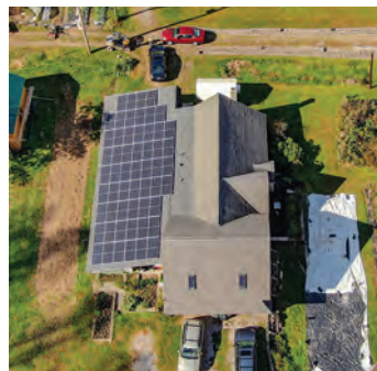
Solar panels generate 20 kilowatts of power at SouthDown Farm. Photo courtesy of Seth Long
