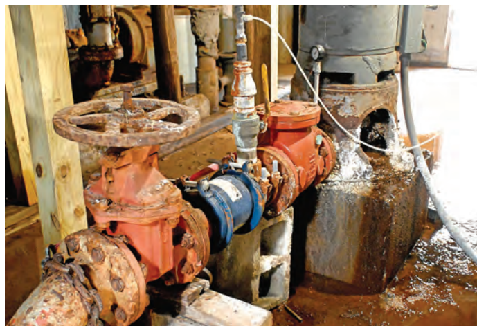
Left, top and bottom: Inside the Kimball water plant in McDowell County, West Virginia, an approximately 60-year-old pump spills water onto a cement floor. The plants serves about 300 customers. Right: Discarded telephone poles hold up the sagging ceiling. Photos by Lorelei Goff
