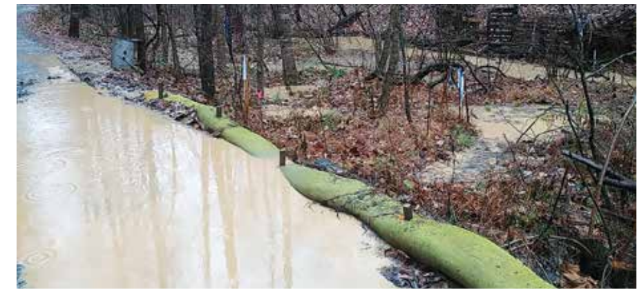
Above, heavy rains on Dec. 1 overwhelmed Mountain Valley Pipeline erosion control measures near Elliston, Va. Photo courtesy of Mountain Valley Watch. At right, a pile of sediment control materials on the side of a steep hill near the same site on Nov. 27. It is close to a tree-sit where pipeline protesters have blocked construction for more than 450 days. Photo courtesy of Appalachians Against Pipelines
