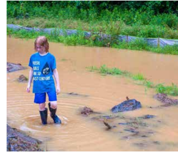
MVP construction at family-owned Four Corners Farm in Rocky Mount, Va., causes significant erosion problems. Photo by Morgan Ashcom
