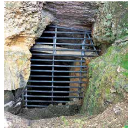
A bat gate blocks a mine entry in Virginia's George Washington and Jefferson National Forest. Photo courtesy of USFS
