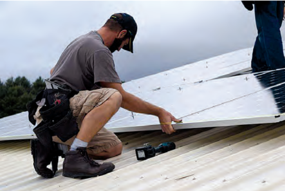
Members of the High Country United Church of Christ congregation installed a 10-kilowatt array of solar panels on the roof of their church on Nov. 6, 2015. Photos courtesy of High Country United Church of Christ
