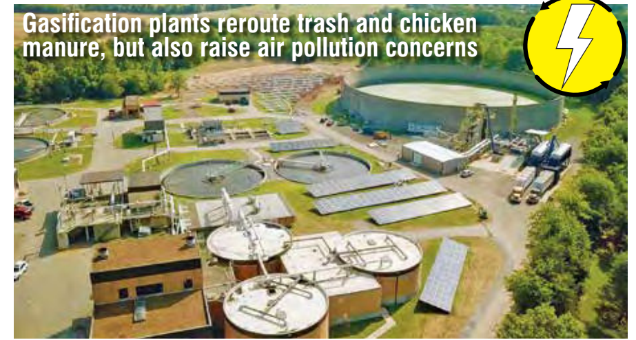
Located in front of the largest circular tank, a gasification plant and solar panels provide two-thirds of the Lebanon, Tenn., wastewater treatment plant's power. Photo courtesy of Aries Clean Energy
