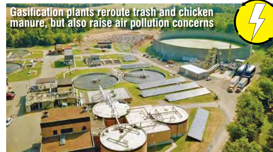
Located in front of the largest circular tank, a gasification plant and solar panels provide two-thirds of the Lebanon, Tenn., wastewater treatment plant's power. Photo courtesy of Aries Clean Energy
