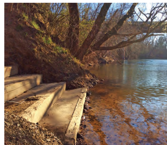
The outlet for the water used to cool a proposed gas-fired power plant would enter the Dan River about 250 feet upstream from the canoe access. Photo by Buck Purgason
