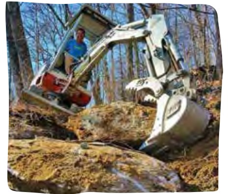
Shrimper Khare positions rocks to armor the trail tread on CMLC's new Weed Patch Mountain Trail. Photo courtesy of CMLC
