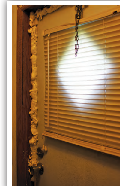
The Wilmoths sealed a door shut to keep air from escaping. Photo by Lou Murrey
