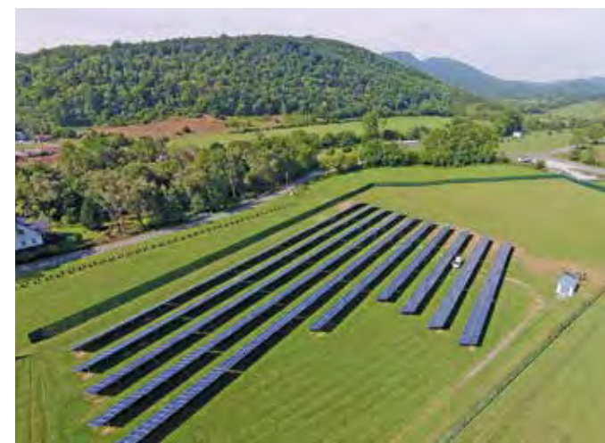
BARC's solar farm contains 1,750 solar panels and produces 550 kilowatts of energy. Photo courtesy of the BARC Electric Cooperative
