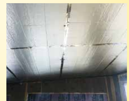
Foil-faced foam boards can reduce heat loss in new or existing homes.
