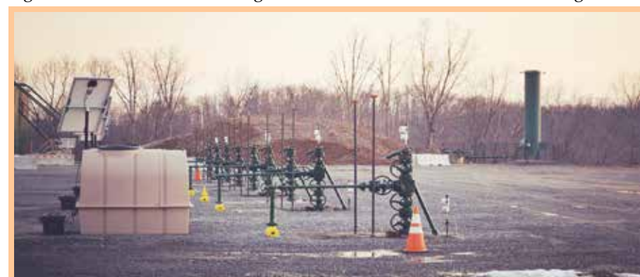
A wellpad site on a split estate in Doddridge County, W.Va., was built by the drilling company to access the minerals beneath the surface owner's land. Photo by Molly Moore
