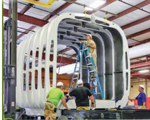
The 3D-printed home and vehicle sit on display at Oak Ridge National Laboratory in East Tennessee. At right, workers assemble the building with components printed on-site. Photos courtesy of ORNL
