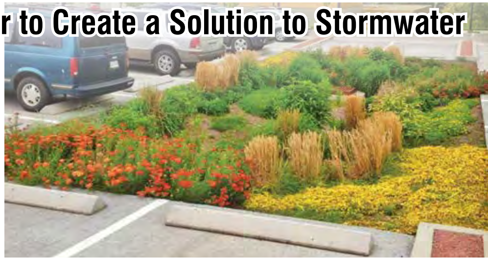
This Renaissance Park Bioretention area in Chattanooga, Tenn., collects water from the parking lot and allows it to infiltrate into the ground. Photo courtesy of the city of Chattanooga
