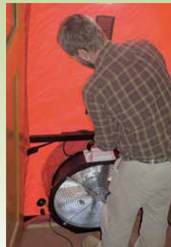
John Kidda, a home energy contractor, prepares a blower door test at Sean Dunlap's home. Photo by Eliza Laubach
