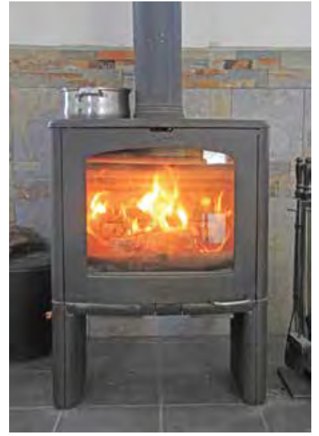
Check for an EPA-certified metal label on the back of a wood stove. If manufactured before 1992, the wood stove is inefficient, says the EPA. Photo by Jamie Goodman
