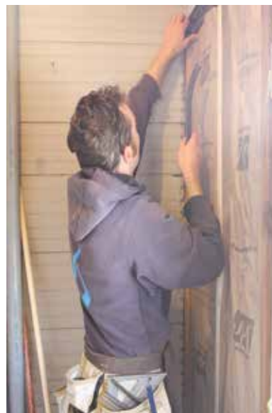
Toby MacDermott replaces a drafty window with an insulated wall. Photo by Sarah Kellogg
