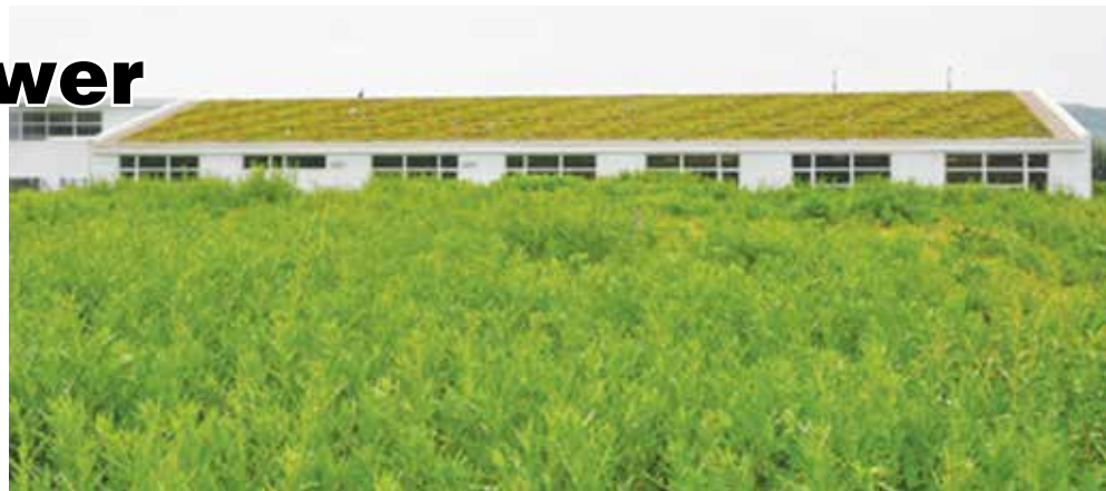
The grounds surrounding the Hocking College Energy Institute in Nelsonville, Ohio, are planted with native grasses that only need to be mowed once per year, and the vegetated roof provides insulation and reduces stormwater flow. Photo courtesy Hocking College
