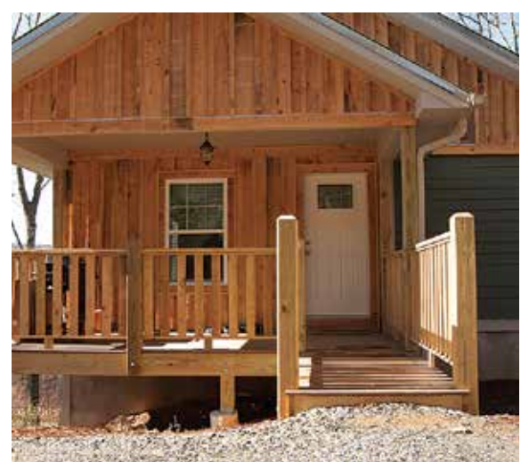
Future homeowners have been working hard with experts and volunteers to construct energy-efficient housing through Watauga County's Habitat for Humanity project. The siding used to construct the GreenWood Community homes, at right, is locally sourced hemlock wood. Photos by Alex Hooker
