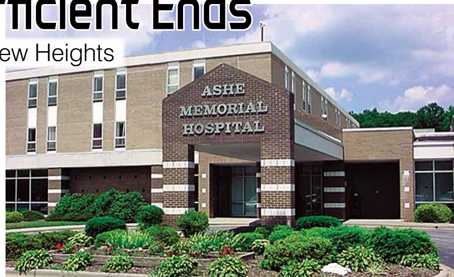
By taking advantage of government loans, a team at Ashe Memorial Hospital in Jefferson, N.C., installed lighting upgrades and energy management tools that save the hospital more than $50,000 each year. Today, Ashe Memorial has reinvested those savings in the hospital, renovating its nursing and birthing centers, and opening a rehabilitation and wellness center. Photo courtesy of Ashe Memorial Hospital
