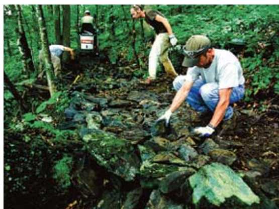
Laying rock by hand for the new trail systems. Photo by Kristian Jackson.
