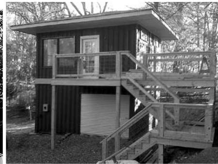
Pictured are Dwellbox's first shipping container construction projects. At top, the small, stand-alone apartment on Hill Street in Boone, N.C. At left, a 1,600 sq ft home called Tad Asana which took three 40' and two 20' containers to construct. The cantilevered design required significantly more engineering than the square apartment building. Photos courtesy of Dwellbox
