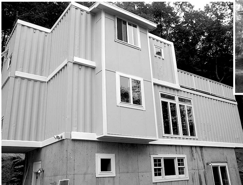
Pictured are Dwellbox's first shipping container construction projects. At top, the small, stand-alone apartment on Hill Street in Boone, N.C. At left, a 1,600 sq ft home called Tad Asana which took three 40' and two 20' containers to construct. The cantilevered design required significantly more engineering than the square apartment building. Photos courtesy of Dwellbox
