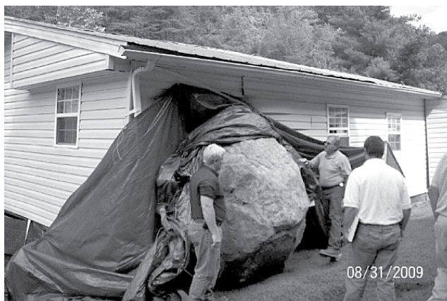
A boulder from a mountaintop removal site crashed into an elderly couple's home in Floyd County, Kentucky. Photo by Lauren McGrath, Sierra Club KY Beyond Coal
