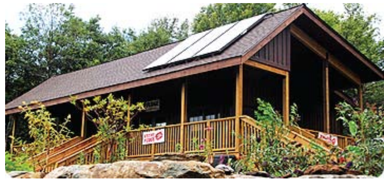
The photovoltaic solar panel on the fudge shop roof is just one example of Grandfather Mountain's green infrastructure. Photo courtesy of Grandfather Mountain
