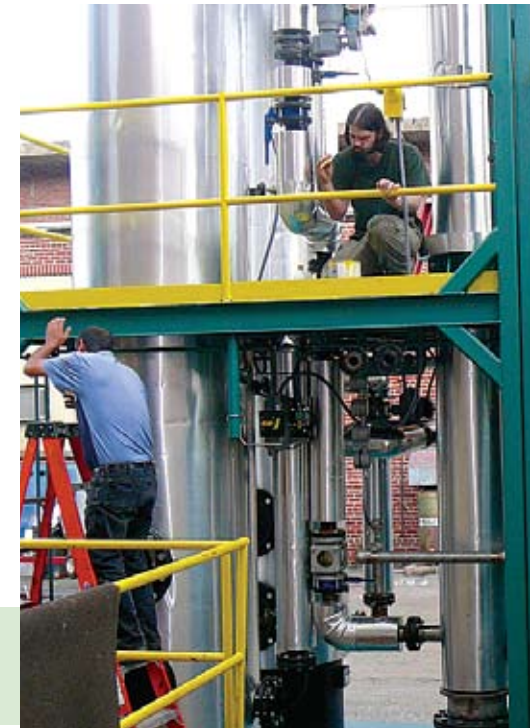
Workers at Pesco-Beam in Roanoke, VA complete work on a molecular sieve. Photo courtesy of Pesco-Beam, www.pescova.com
