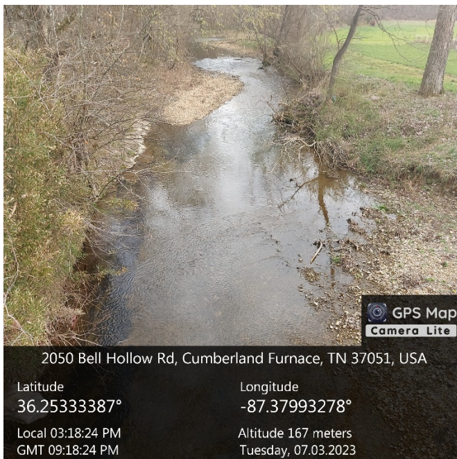
Figure 6. This was taken from the bridge at 2050 Bell Hollow Rd., looking upstream of Furnace Creek toward the area that would be crossed by the pipeline. This stream is an important resource for several farmers and local wildlife.
