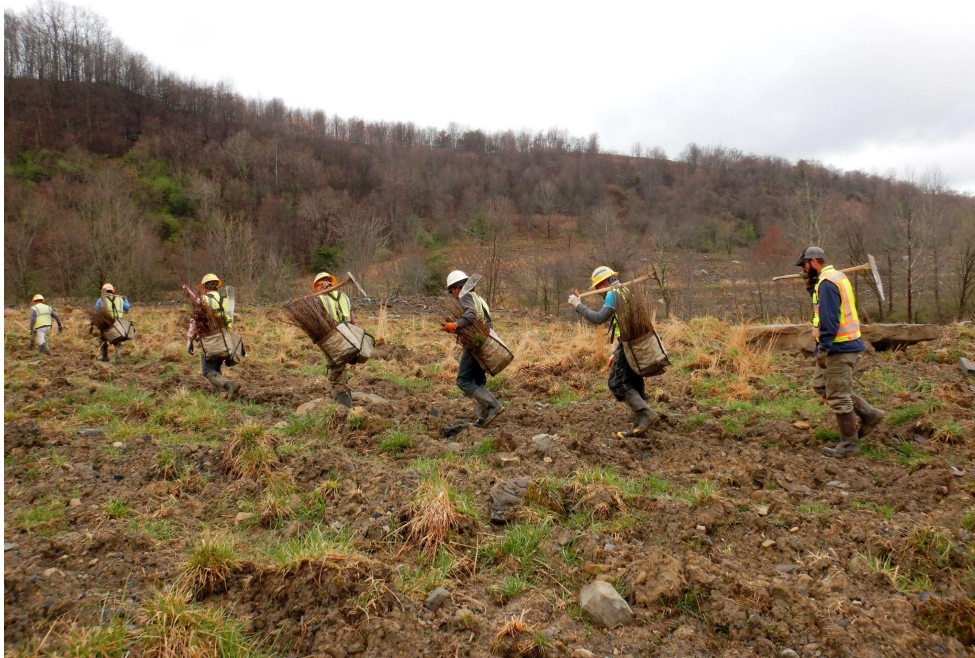
Professional tree planters hike over ripped ground to begin planting trees at the Mammoth 22 project area in West Virginia, the site of a former mine. Photo courtesy of Green Forests Work.
